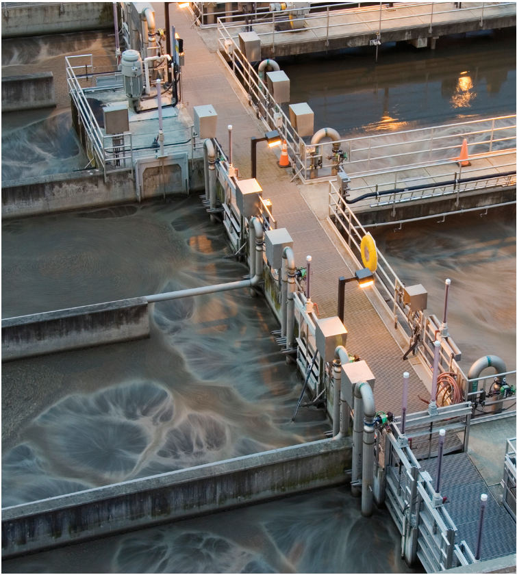
Aeration tanks use bubbling air to help suspend microorganisms in the wastewater. These microorganisms can then break down waste materials into carbon dioxide and clean water.
