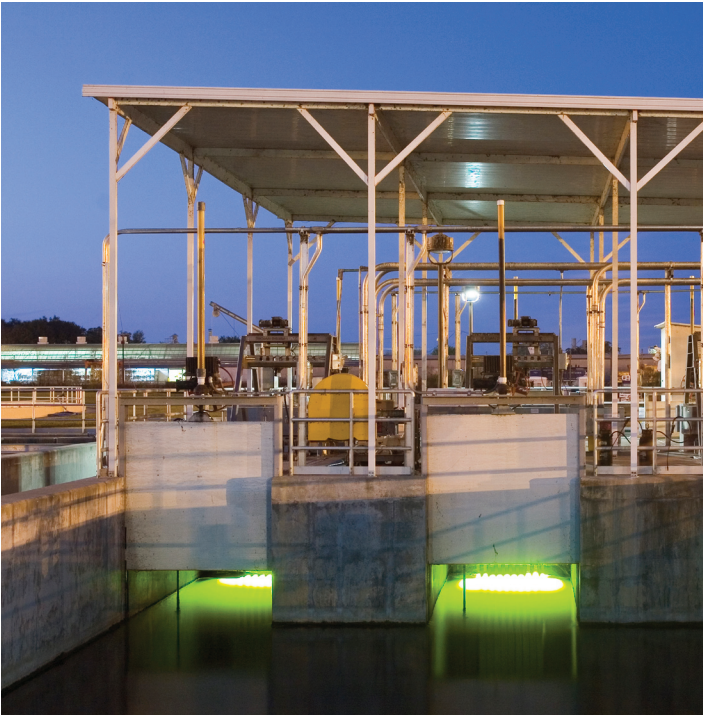
As a final step in the treatment process, water can be disinfected through exposure to UV light. Running the water over these lights can quickly kill any remaining pathogenic bacteria.
