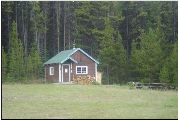
Jack Shack – overnight accommodation for 12 people, 200 m from the trailhead.
